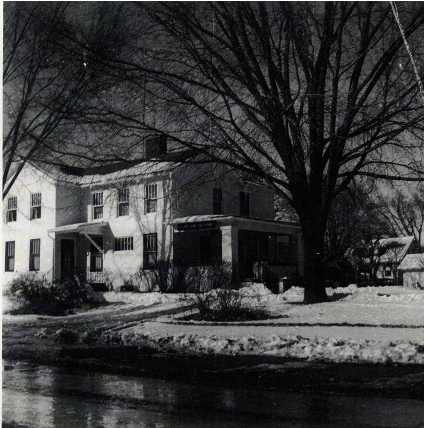
Taylor Funeral Home , Brimfield, IL c. 1955. Copy of original photo provided by Jane Taylor Becksted.
